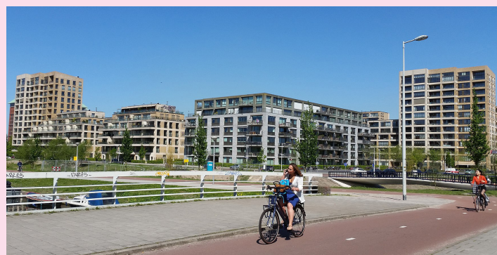
Amsterdam New West district contains around 40,000 households of which 10,000 are served by a new smart grid. The area is characterised by a high penetration of smart meters and the largest number of solar panels in Amsterdam 9 . The smart grid has delivered a number of key benefits including: reduction in the frequency and duration of power outages; increased capability to accommodate E-mobility; facilitate active participation from sustainable energy suppliers and has avoided sharp increases in the price of electricity transmission.
